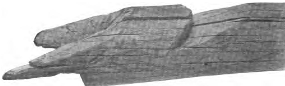
FIG. 80. LOWER END OF RAFTER.
